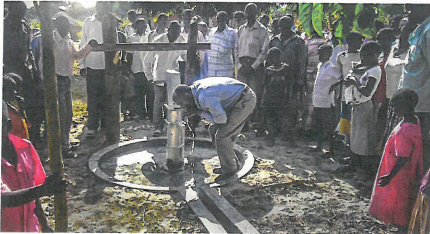
Building a well in Uganda.
